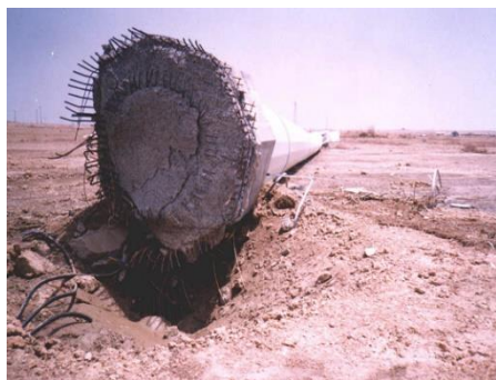
Figure 4: Foundation failure due to design and construction defects
