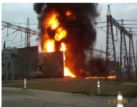
Figure 5: Substation fire caused by construction defect
